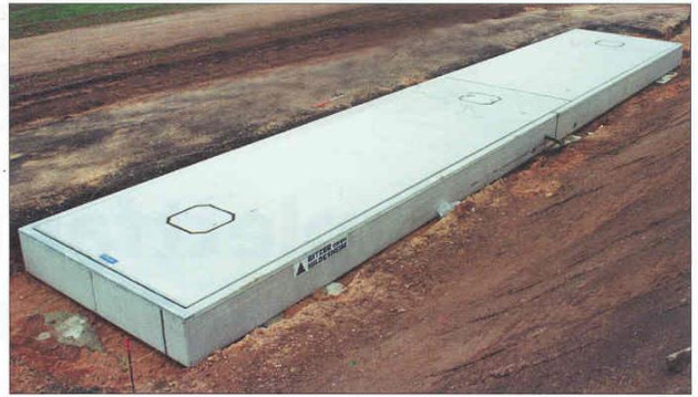
Installation of plant-assembled scale
